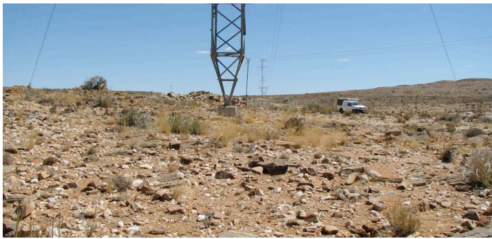
Figure 6. Minimal disturbance in the vicinity of a tower on an existing transmission line.
