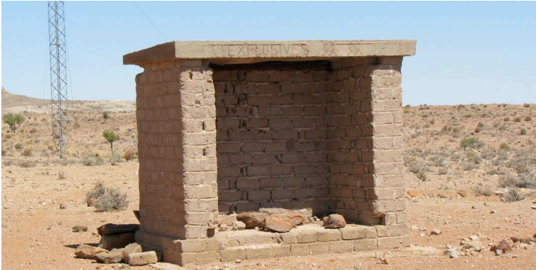
Figure 5. Remains of pre-1961 mining infrastructure.
